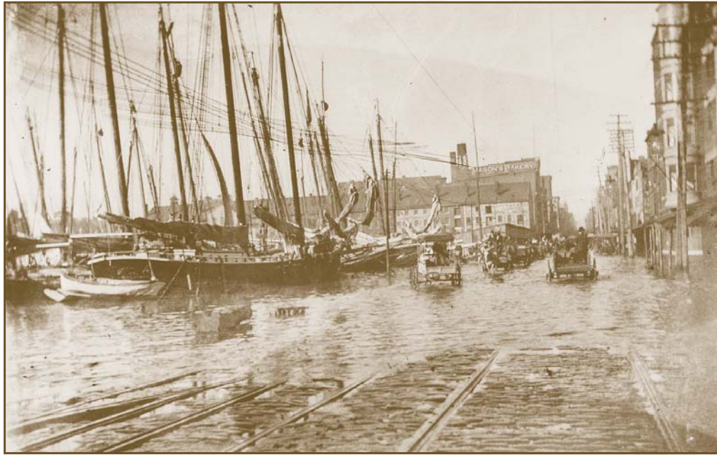
Pratt Street flooded.
